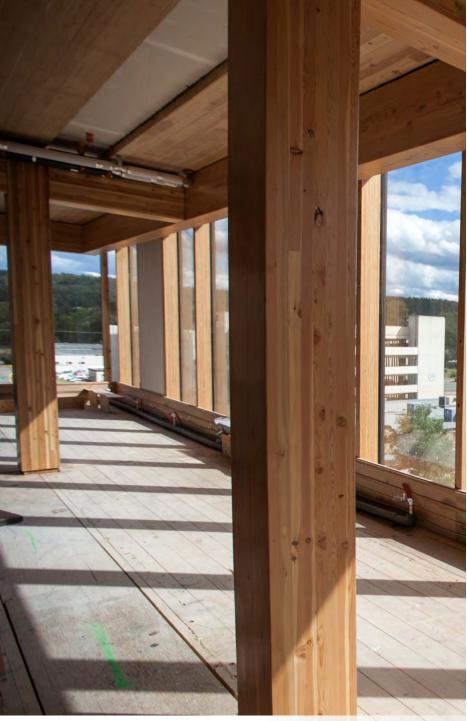
Glulam posts supporting mass timber beams of the Wood Innovation and Design Centre
