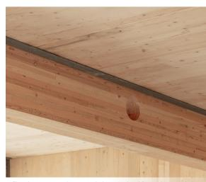
Floor beam supporting mass timber panels with openings for plumbing, electrical cables and other connections.
